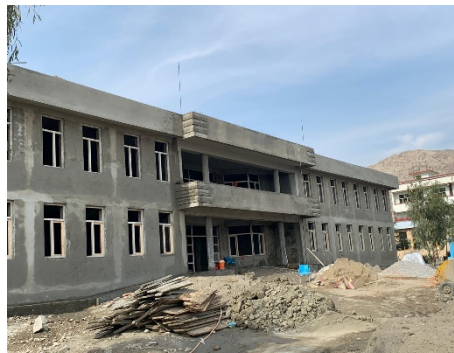
View of Daman middle school being built by UNHCR. © UNHCR/ Eamal
