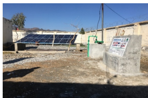
UNHCR dug bore well and provide Solar system to Abdul Shakur boys school to solve their water challenge/PARR-Mirwais Mina-PD#07/Iqbal Ferahmand-Liaison Officer
