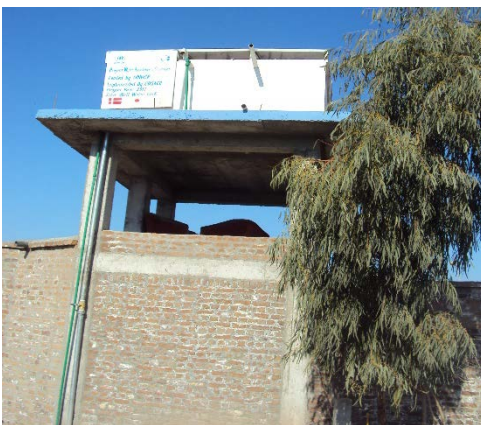
View of the water reservoir constructed by UNHCR in SMNT@ UNHCR/ Eamal
